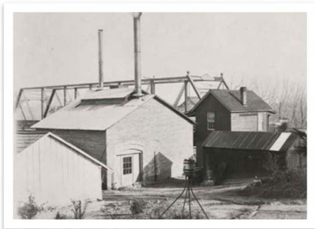
Historical photo of worksite located at 600 Rio Street. Source: PG&E
